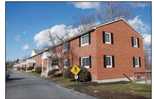
Above (top to bottom): Cluster subdivision along Angelo Drive (RA-3 District); single-family detached homes on Pine Court (R-2 District); and garden apartments within the RM-1 Multi-family District.
