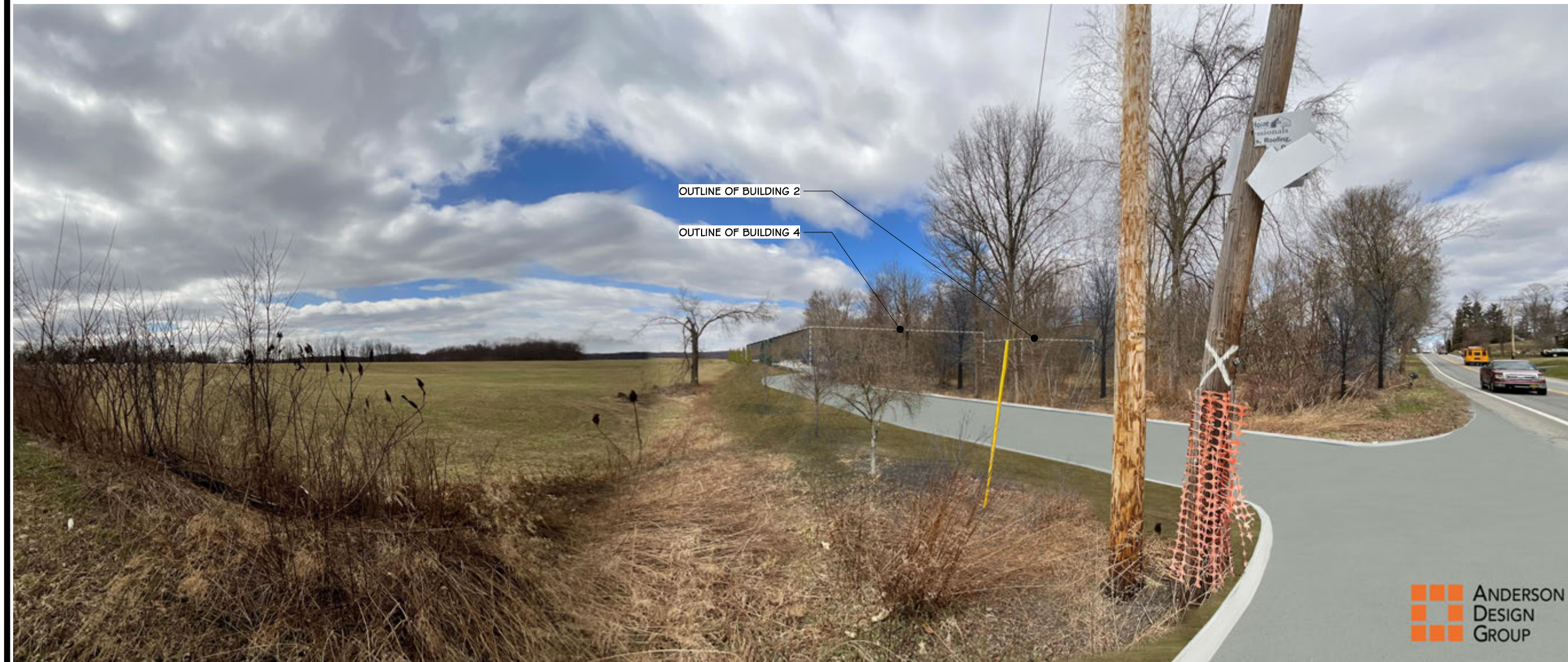
② PROPOSED VIEWSHED FROM UNION STREET (VANTAGE POINT 3) ENTRANCE - 35' HT. COMPARISON LANDSCAPING AT YEAR 1
